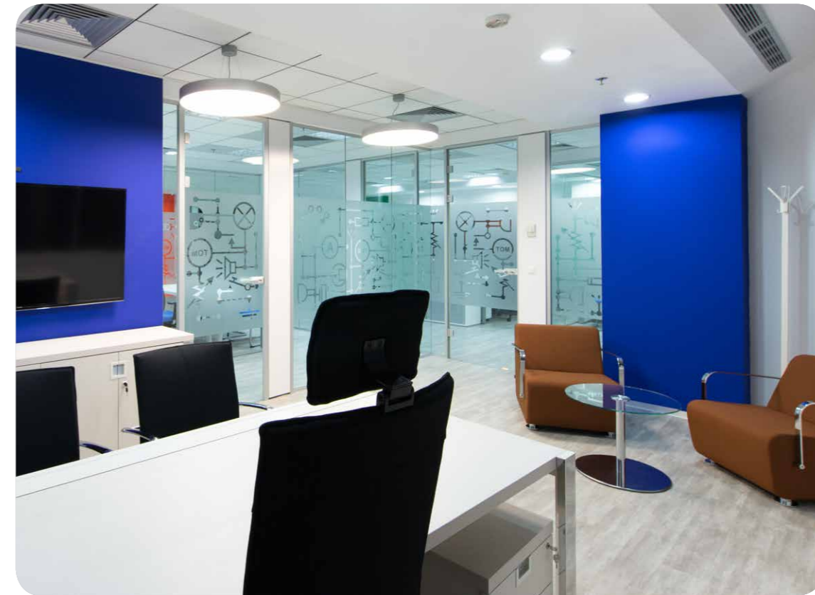
Single glazed glass partition Sky30 system, with technical module and single glazed doors
