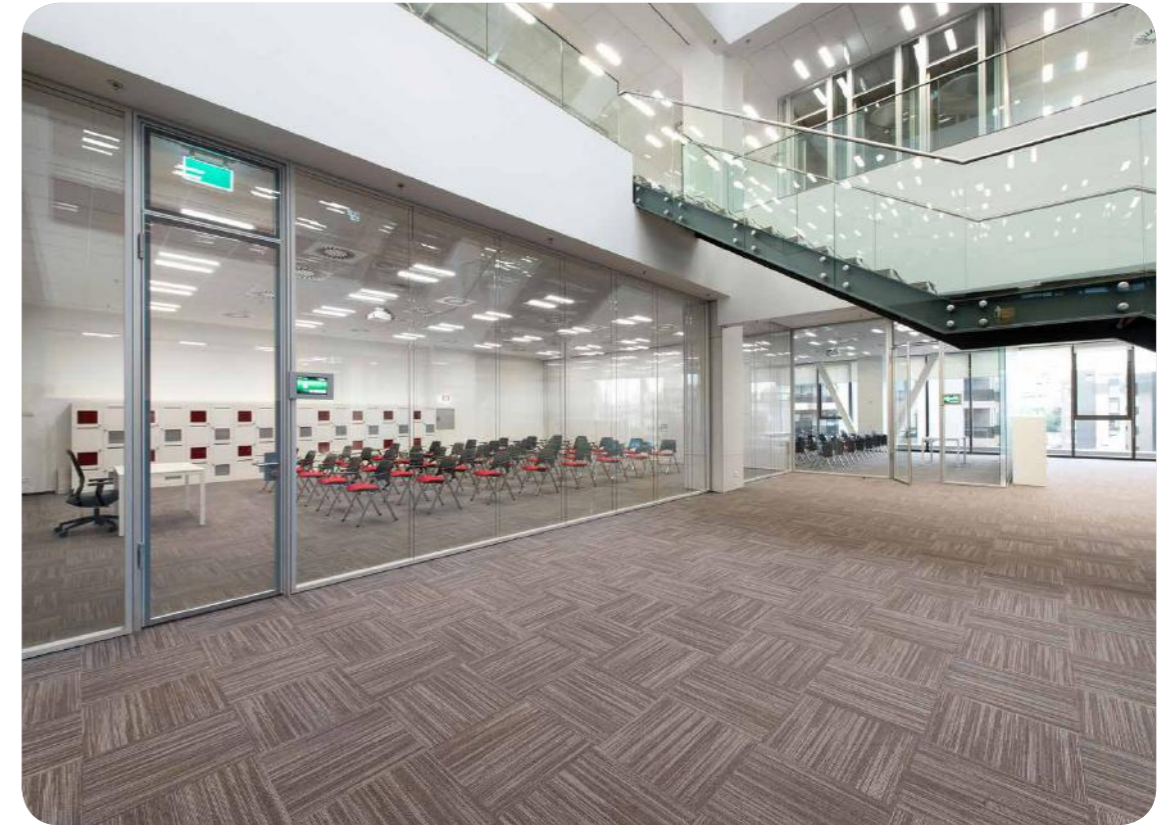
Double glazed Vitrum V10 system with DG double glazed door
