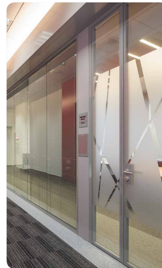
DG double glazed glass door with technical panel and V10 system
